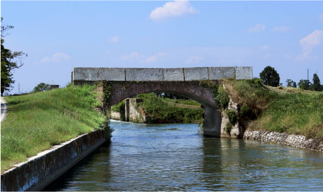
BRIDGE SITE PHOTO
